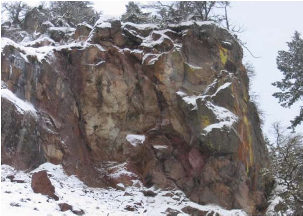
ROCK SLOPE AFTER ROCKFALL EVENT FROM UPPER ROAD
