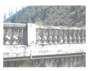
**Figure 5:** Balustrade on Rogue River (Rock Point) Bridge, 1920, illustrating urnshaped balusters *Source:* Author
