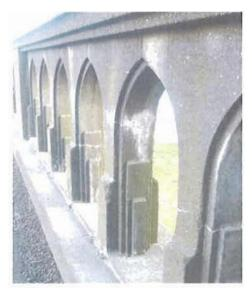
**Figure 30:** Balustrade at Yaquina Bay Bridge, 1936, illustrating Gothic arch opening framed by Art Deco setbacks *Source:* Author
