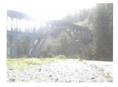
Figure 16: Substructure of Cape Creek Bridge, 1932, illustrating parabolic deck arch and tiers of columns
