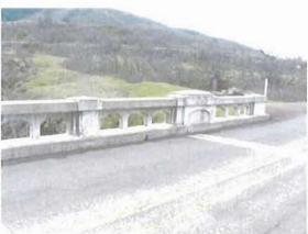
**Figure 6:** Balustrade on Dry Canyon Creek Bridge, 1921, illustrating segmental arch design
