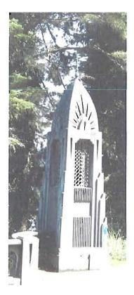
Figure 21: Primary entrance pylon at Siuslaw River Bridge, 1936, illustrating metal grate and sunburst motif
