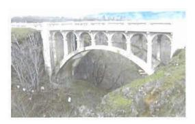
Figure 9: Dry Canyon Creek Bridge, 1921, illustrating open-spandrel deck arch design
