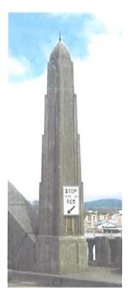
Figure 22: Secondary entrance pylon at Siuslaw River Bridge, 1936, illustrating incorporation of setbacks *Source:* Author
