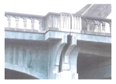
**Figure 44:** Detail of Big Creek Bridge on US 101, 1931, illustrating difference in coloration and texture of bridge fabric where cathodic protection was applied *Source:* Author
