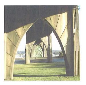
**Figure 29:** Substructure of Yaquina Bay Bridge, 1936, illustrating Gothic arch opening in the supporting bents framed by Art Deco setbacks *Source:* Author
