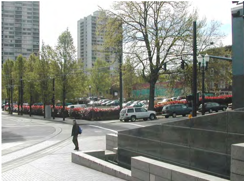
Existing view of Block 153 [Jasmine] from Urban Center Plaza
