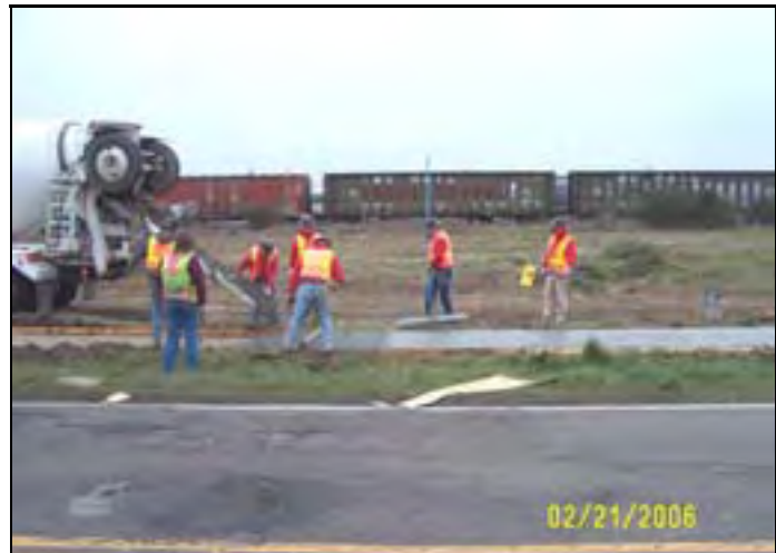
New street capacity under construction.
