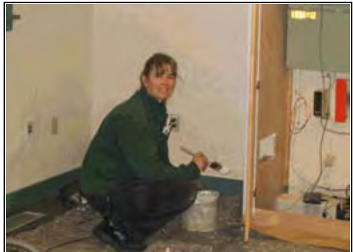
Interior painting at River House
