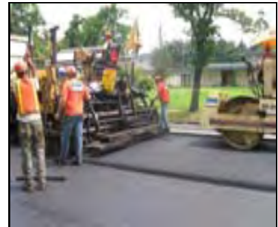
Capital pavement overlay project in progress.
