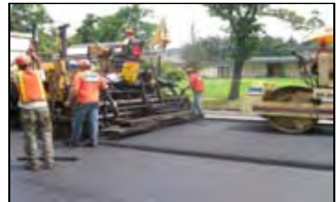
Capital pavement overlay project in progress.
