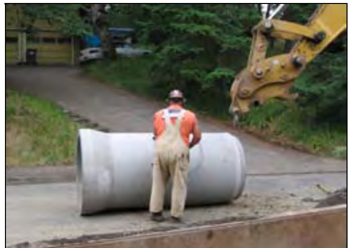
Installing stormwater pipe
