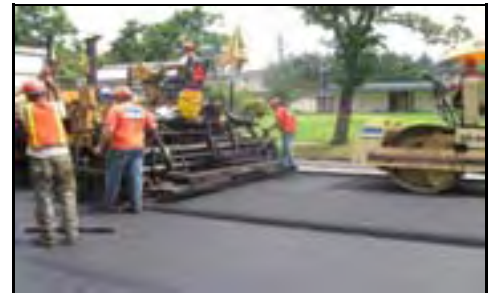
Pavement Preservation Program in action.
