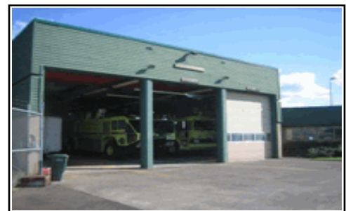
Current Eugene Airport Fire Station
