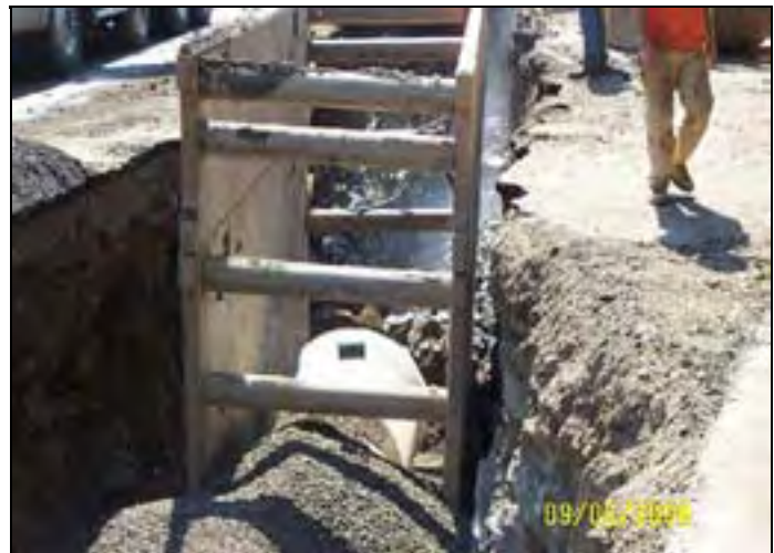
Stormwater line construction underway.
