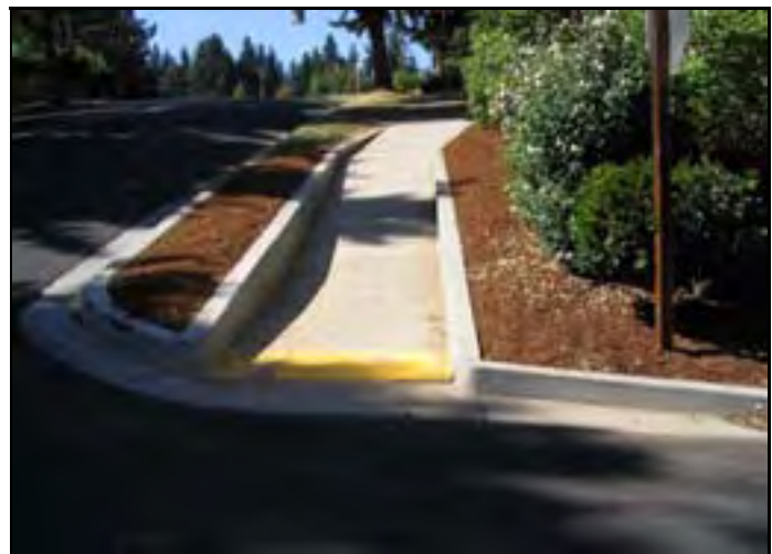
Accessible sidewalk ramp
