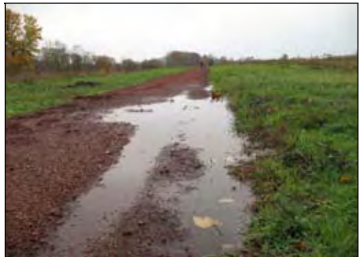
Failing park irrigation system.
