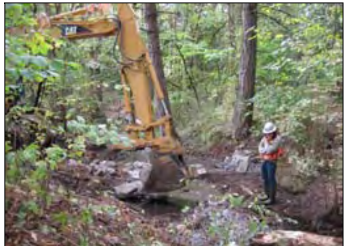
Streambank stabilization work.
