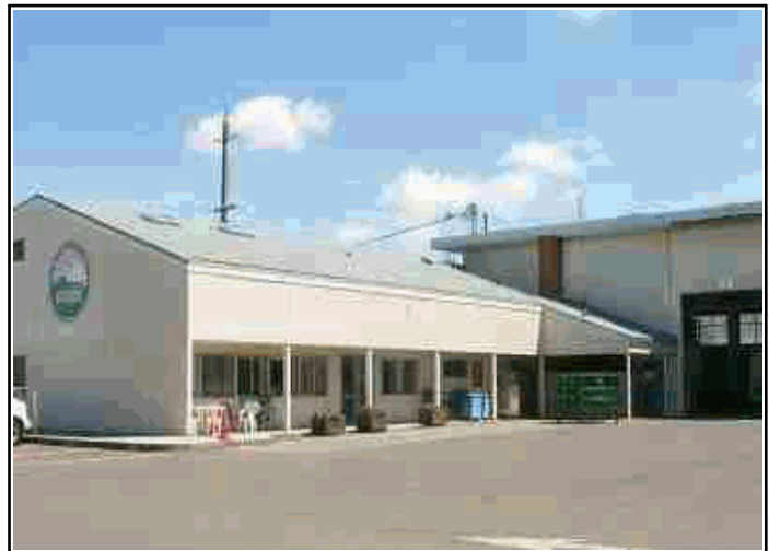
Current Fleet Maintenance facility.
