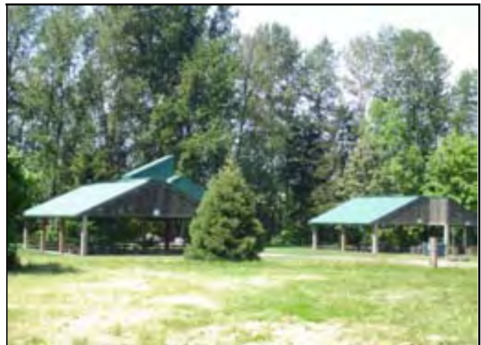
Area around Alton Baker Park picnic shelters in need of renovation.
