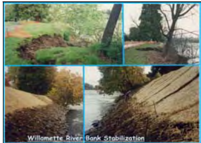
Willamette river bank stabilization
