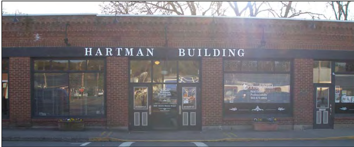
e. Hartman Building: 210 S Water St
