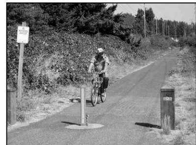
Bollards slow cyclists and prevent vehicles from entering the trail.
