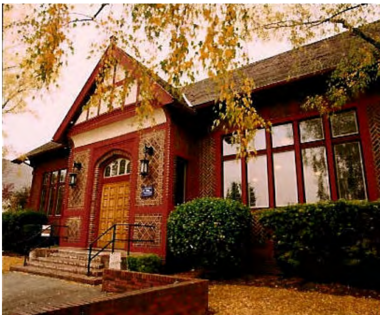
Gresham Carnegie Library Figure 1
