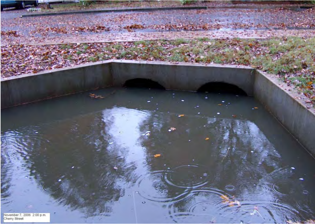
Cherry Lane Culvert - Estimated depth from crown elevation to WSE is 8".
