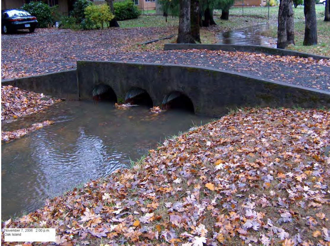
Culvert C (L17) – Estimated depth from crown elevation to WSE is 14”.
