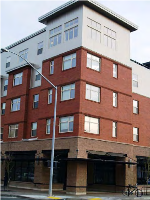
Royal Building, Springfield
