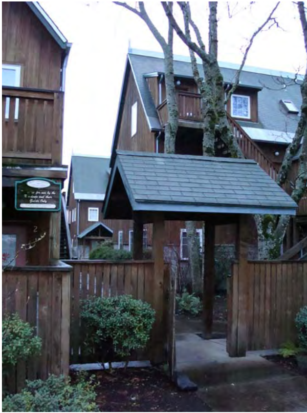
Multifamily housing – Eugene, OR. This student housing complex at the University of Oregon represents well designed units at increased density.
