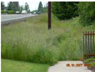
Discontinuous and Below Grade
