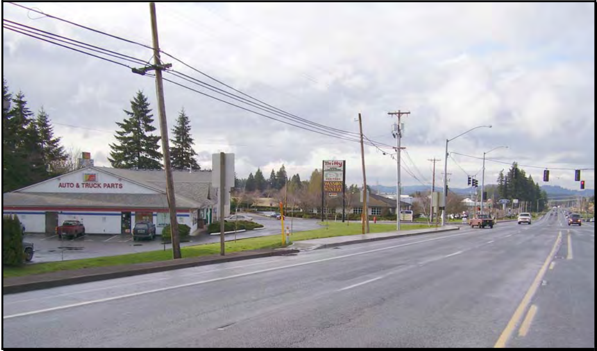
Photo 6-1A: US 26 Westbound approaching Ruben Lane - Existing Condition
