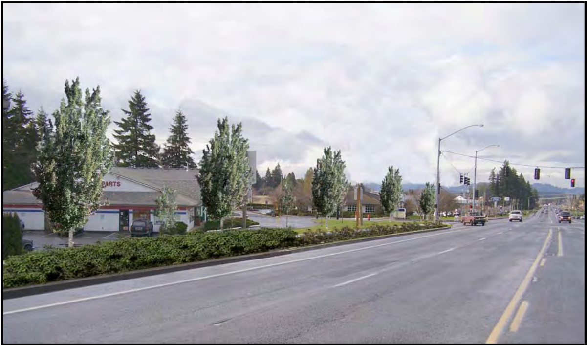
Photo 6-1B: US 26 Westbound approaching Ruben Lane - Fully Improved
