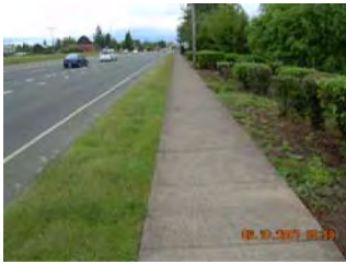
Typical Uncurbed Sidewalk
