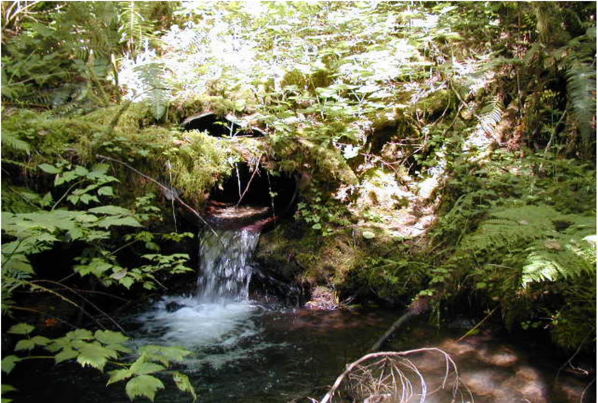
Figure 1: Fish passage barrier in the McGowan Creek Watershed
