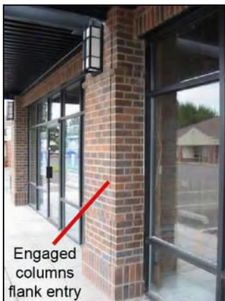
Figure 43 Entry flanked by engaged columns and lighting
