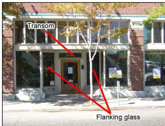
Figure 38 Example of entry with transom and flanking glass
