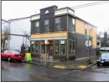
Figure 32 Top of building features a parapet
