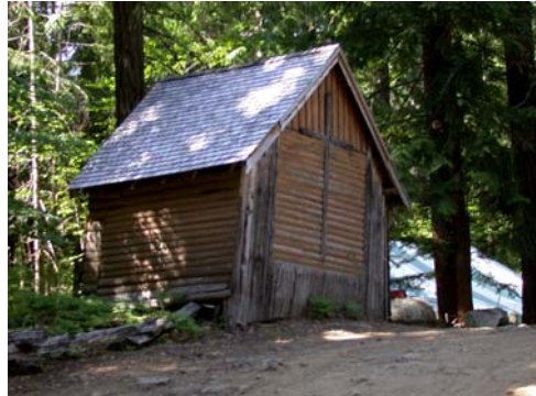
Wood shed south and east elevations
