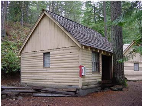
Cabin #2/Birch west elevation and south facade.
