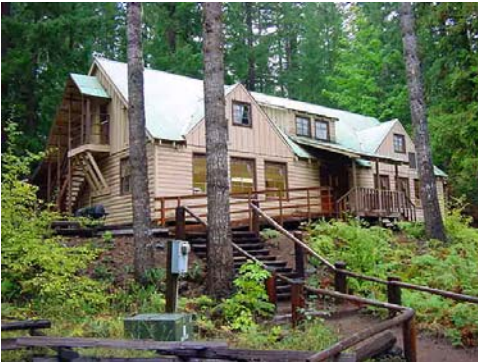
Mess Hall/Dormitory southwest elevation and southeast facade.
