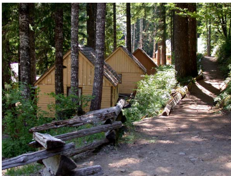
The oldest dormitory cabins dating from ca. 1949, looking west.
