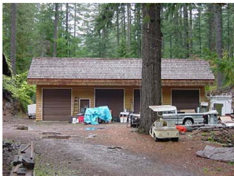
Shop/Storage Building east facade, looking west.
