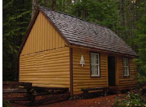
Cabin #6/Fir east elevation and north facade.
