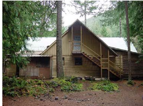
Mess Hall/Dormitory northwest (rear) elevation.
