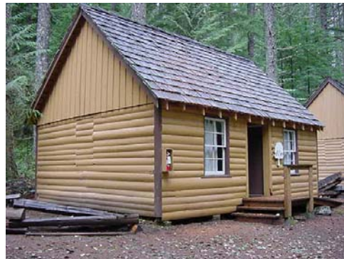
Cabin #5/Elm east elevation and north facade.
