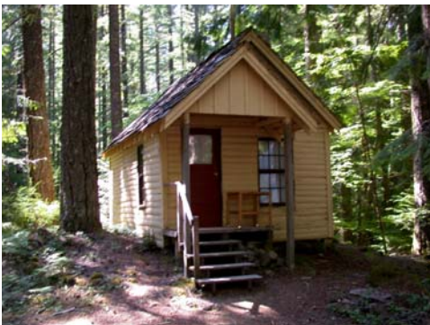
Cook's Cabin/Guest Cabin south elevation and east facade.
