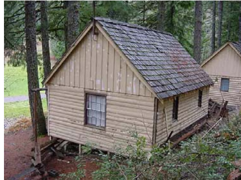
Cabin #1/Alder east and north elevations, demonstrating typical cabin rear.
