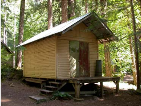
Generator House/Lifeguard Cabin north elevation and west facade.
