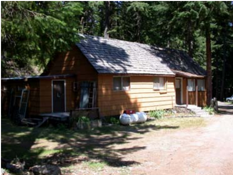
Caretaker's Cabin/Assistant Manager's House west elevation and south facade.
