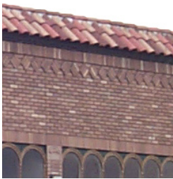
Terra cotta and brick
