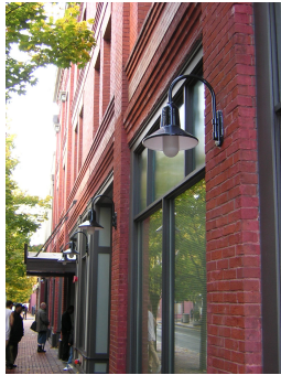
Building lighting and transom windows
