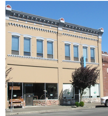
Unified elements and a strong, tri-partite structure can strengthen a building's (and a downtown's) overall image
