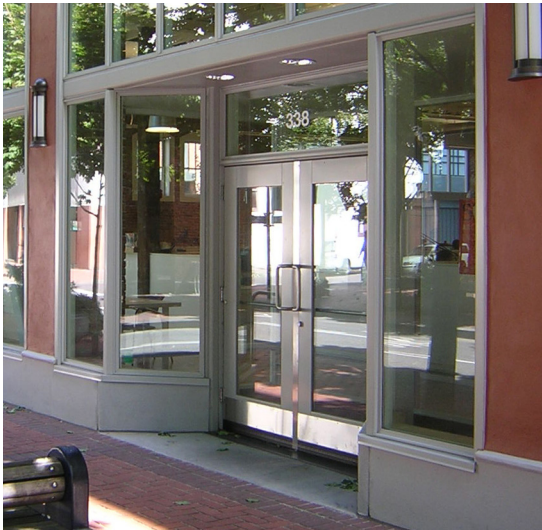
Prominent, recessed entry that features transom windows, large glass entry doors, and flanking windows.
