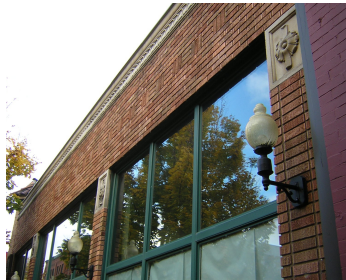
Building lighting, medallions, and transom windows
