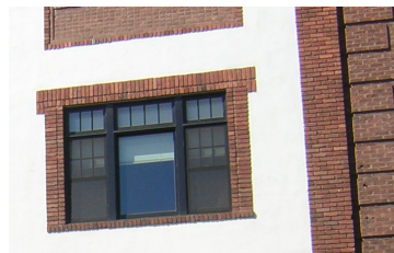
Stucco and brick
