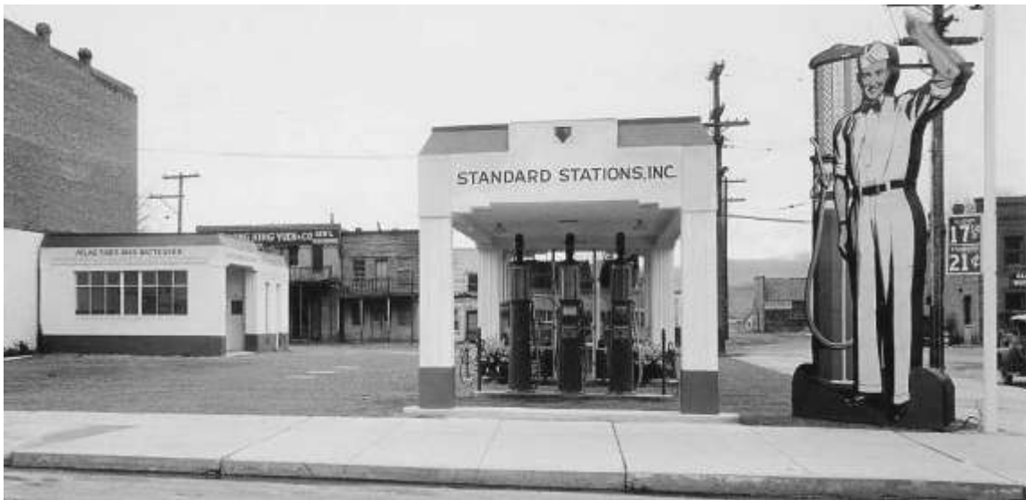
Standard Station at the corner of Auburn Avenue and Main (formerly Front) Street looking east ca. 1930. The Wing Hing Yuen store is seen in the middle, left of the photograph, partially obscured by the Standard Station garage. Source: Baker County Library, Baker City, Oregon, Record 1992.11.
