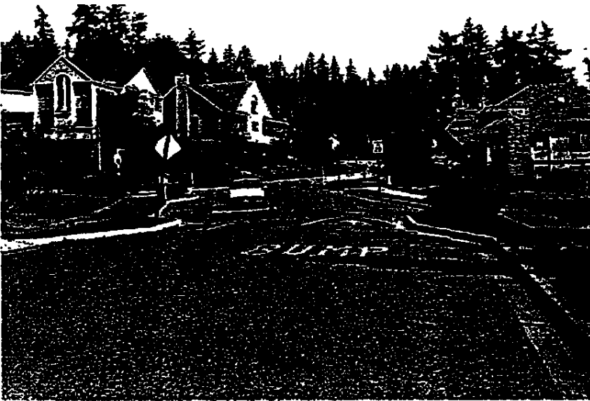
Figure 5-2 Visibility is a key design issue at an RTM device
