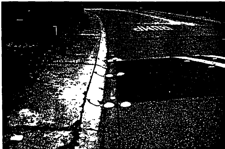
Figure 5-1b. Speed Hump Edge Treatment
