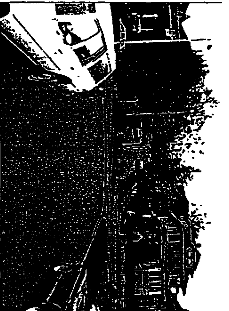
FIGURE 3 Turn lane cut into partial diagonal diverter E. Highland Ave. at 18th Ave., Seattle, Washington
