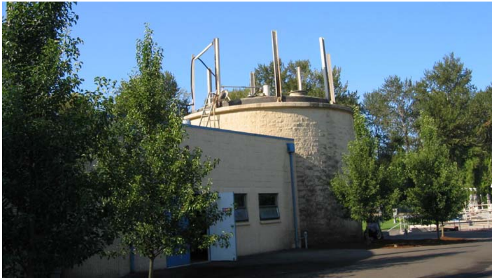
Figure 9-15. Silverton Anaerobic Digesters and Digester Control Building
