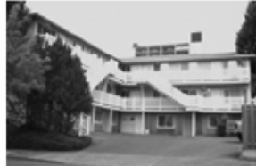
Apartment building at N. Edison and Baltimore
