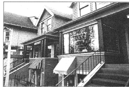
Mary Munly Houses #1 & #2 (l - r), 720-722 NW 23 rd Avenue
