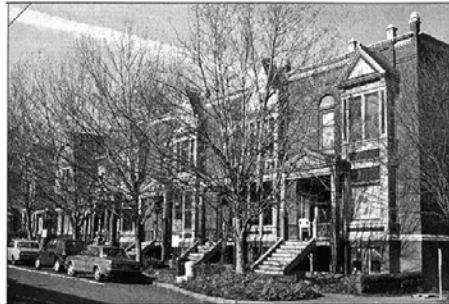
The Campbell Townhouses, 1705 - 1719 NW Irving Street
