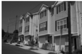
Rowhouses at N. Burlington and Willamette
