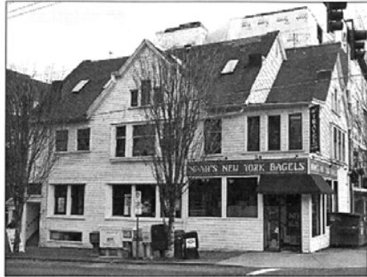
Wilfred & Gustav Burkhardt Building, 500-510 NW 23 rd Avenue
