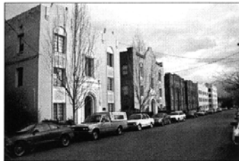
Looking northeast along NW Irving, between NW 19 th & NW 20 th Streets
