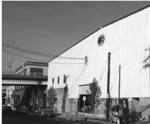
Industrial building that uses concrete exterior at the street level and metal above.
