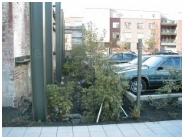
Recommended: Polluted water runoff from parking lot is mitigated by a landscaped swale (NW 10th and Irving, Portland)
