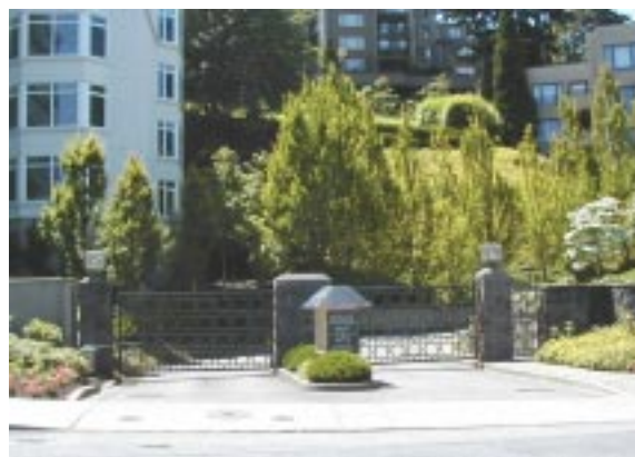
Not Recommended: Private compounds (NW Westover, Portland)
