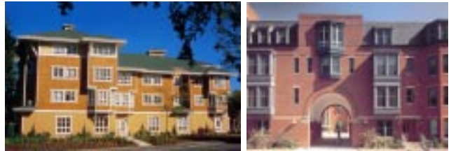
Recommended: Boldly articulated facades benefit from the inclusion of medallions, belt courses, varied cladding materials or other surface articulation (SW Yamhill and 4th, NW Hoyt and 12th, Oakland, CA, Boston, MA)
