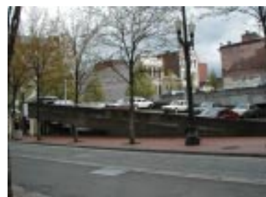
Not Recommended: Exposed sloped parking structure (SW Morrison and 1st, Portland)
