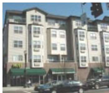
Not Recommended: Bays that are poorly detailed, clad with corrugated metal, or include projecting mechanical units (Salem Transit Center, Union Station Housing, NE Weidler and 15th, Union Station Housing)
