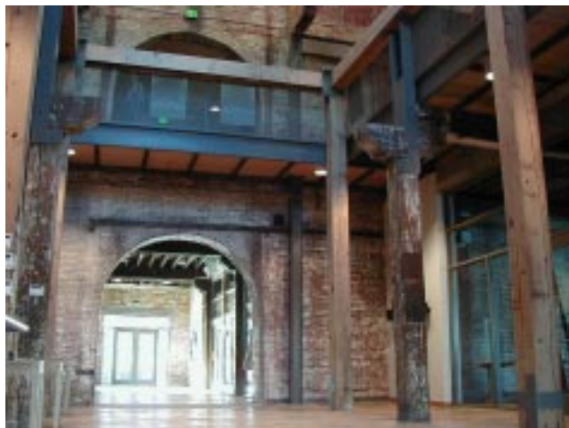
Recommended: Use of salvaged and recycled materials (NW 10th and Irving, Portland)
