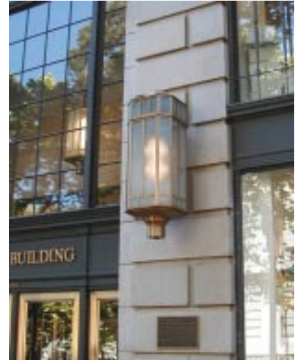
Recommended: Decorative wall sconce designed as part of overall building facade composition (SW Yamhill and 5th, Portland)
