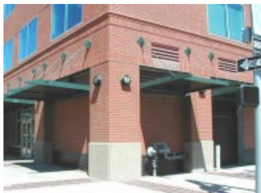
Not Recommended: Unwelcoming blank walls at building corner (Salem)
