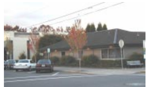
Not Recommended: Main Street commercial building that differs radically from its neighbors in form and mass (Downtown Milwaukie)
