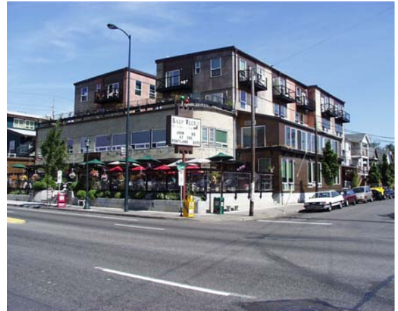
Restaurant and Shops with Apartments
