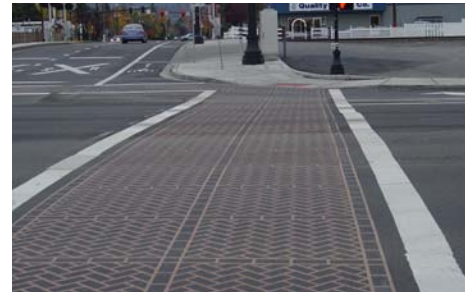
Enhanced crossing markings
