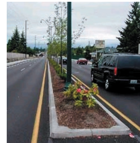
Adding a landscaped median to an existing wide street can be achieved within 6’ of roadway. (Bend)
