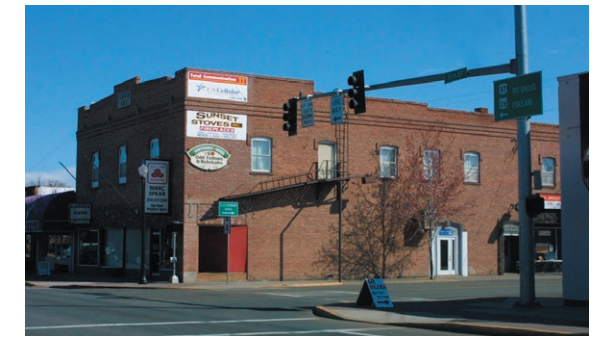
The IOOF Building at 5th and D, which is the “100% corner”, the heart of Madras’ commercial area.
