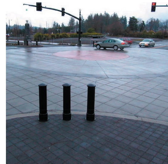
This intersection in Lake Oswego has been repaved, creating a signature gateway, slowing car traffic and making pedestrian crossings safer. Note the bollards separating the roadway from the sidewalk.
