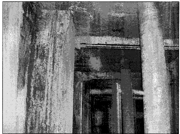
LOOKING NORTH @ ROUND COLUMNS
