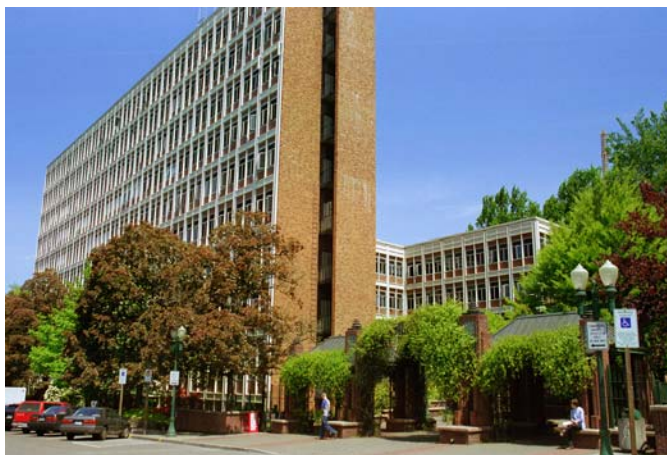
Figure 4.47. PLC from Kincaid St. Photograph by Byoung-Wook Jun
