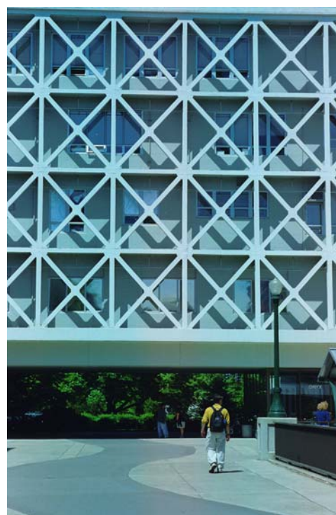
Figure 4.48. Steel Structure of Onyx Bridge Photograph by Byoung-Wook Jun
