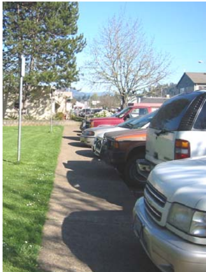
Example of walkway overhang
