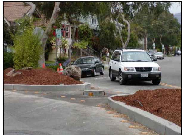
Diverter in Berkely, CA Allowing Emergency Vehicle Access
