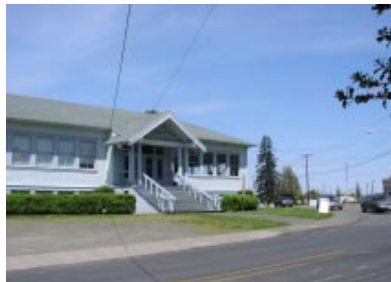
City-owned schoolhouse parcel at North Sherwood Boulevard and 3 rd Street
