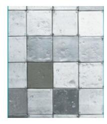
RECYCLED METAL TILES ARE MADE OF 100% RECYCLED ALUMINUM OR BRASS. INSTALLATION IS SIMILAR TO OTHER TILE, USING MORTAR AND GROUT TO BOND TO WALL SURFACE.
