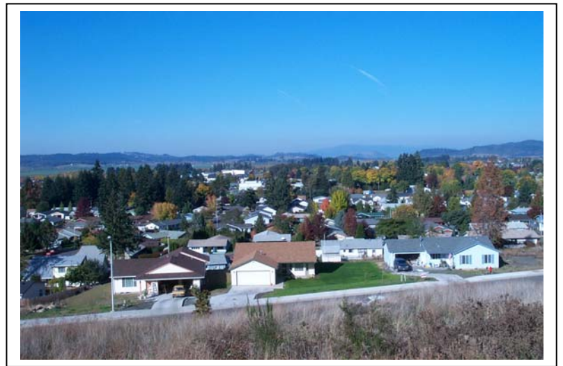
City of Creswell (looking north)
