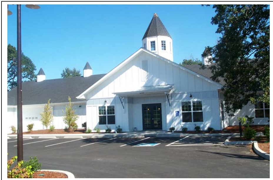
Newly constructed South Willamette Veterinary clinic
