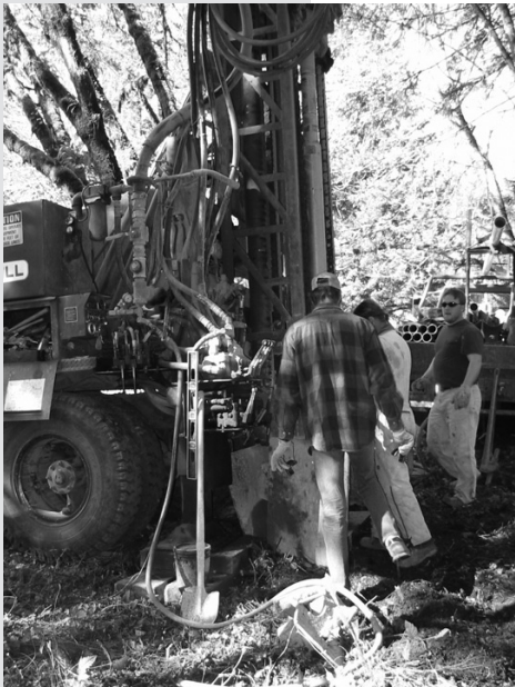
Courtesy of Wren Community Hall and Corvallis Well Drilling
