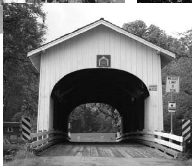
Harris Covered Bridge
