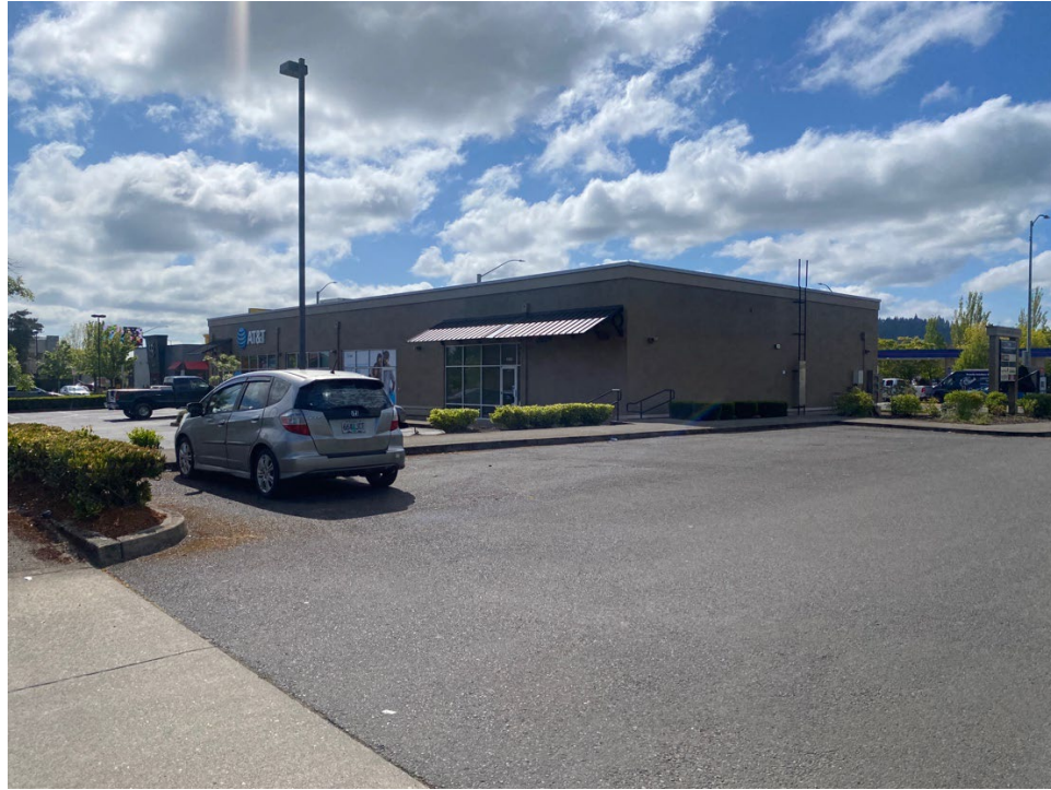
Figure 10: Image of part of the unmarked parking along the back of the Target parking lot.
