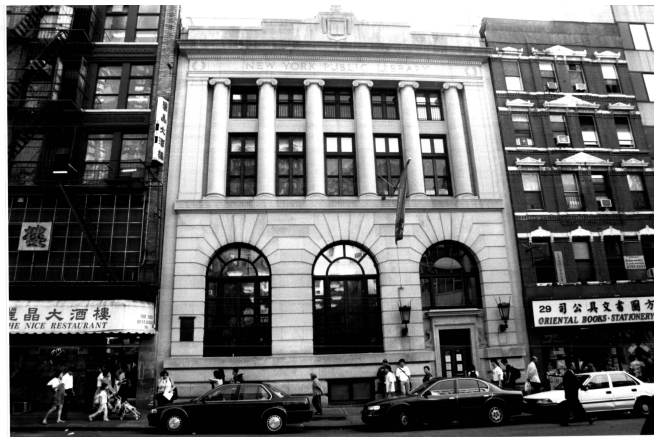
Image 1: New York Public Library Chatham Square Branch Exterior
