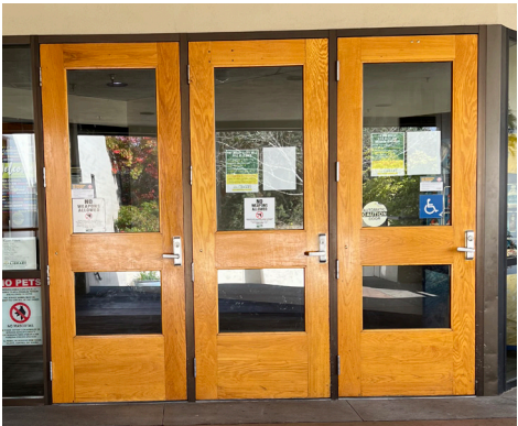
Image 35: Main entry door to Springfield Public Library. Springfield City Hall is also accessible through this entrance.
