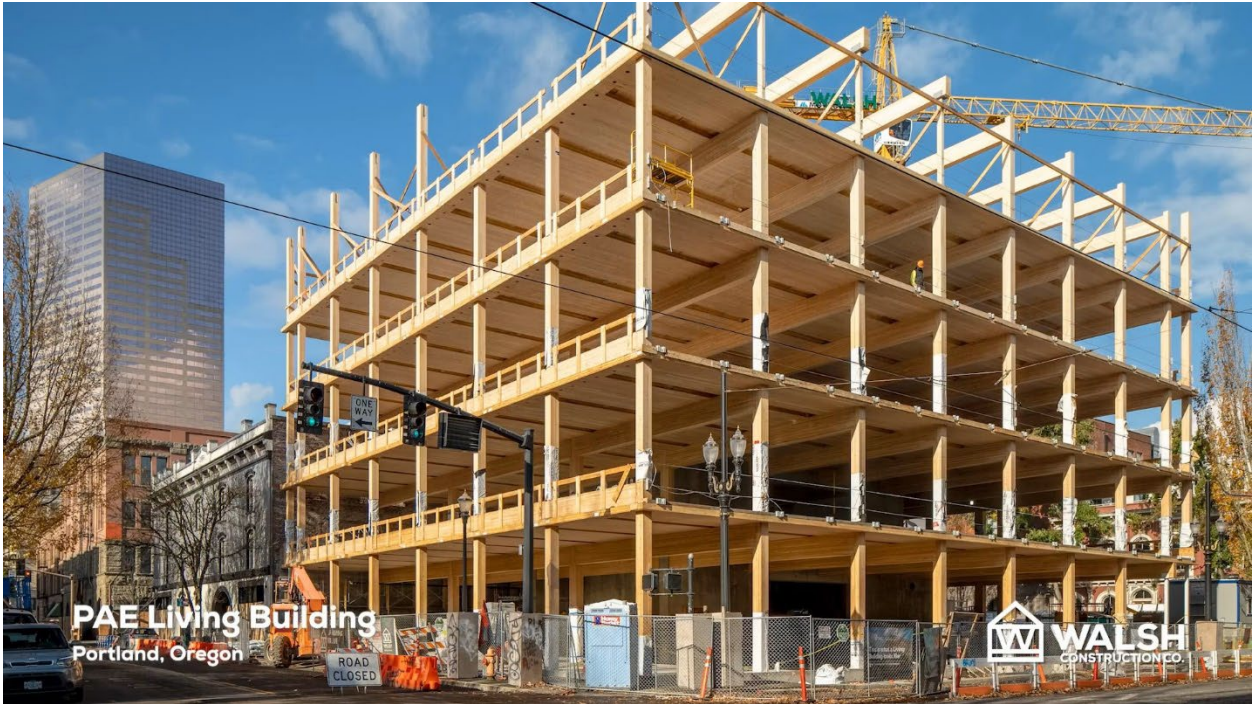
Figure 9. PAE’s building construction, showing CLT framing, courtesy of Walsh Construction Co.
