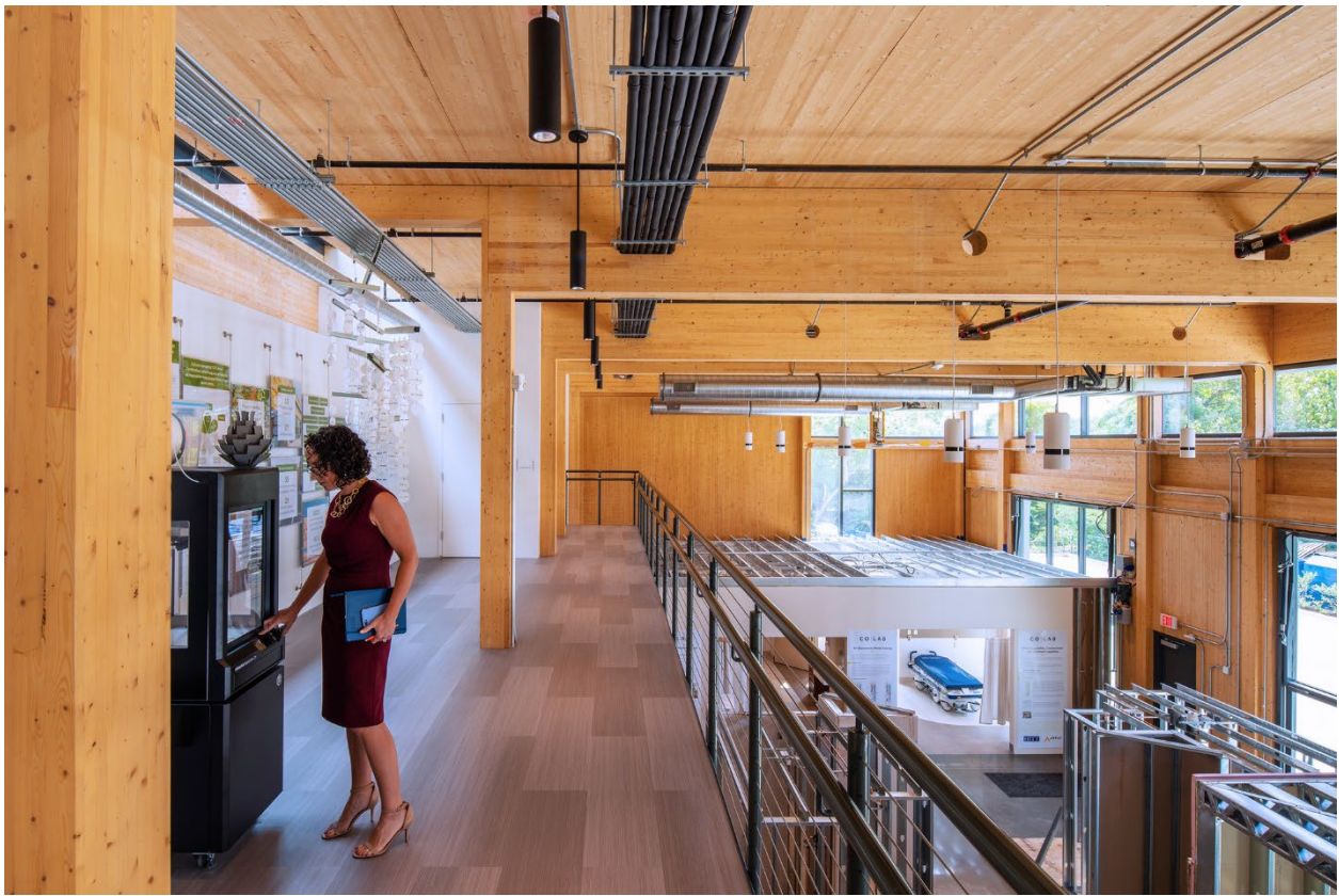
Figure 11. Co | Lab's CLT and glulam, courtesy of ArchDaily.
