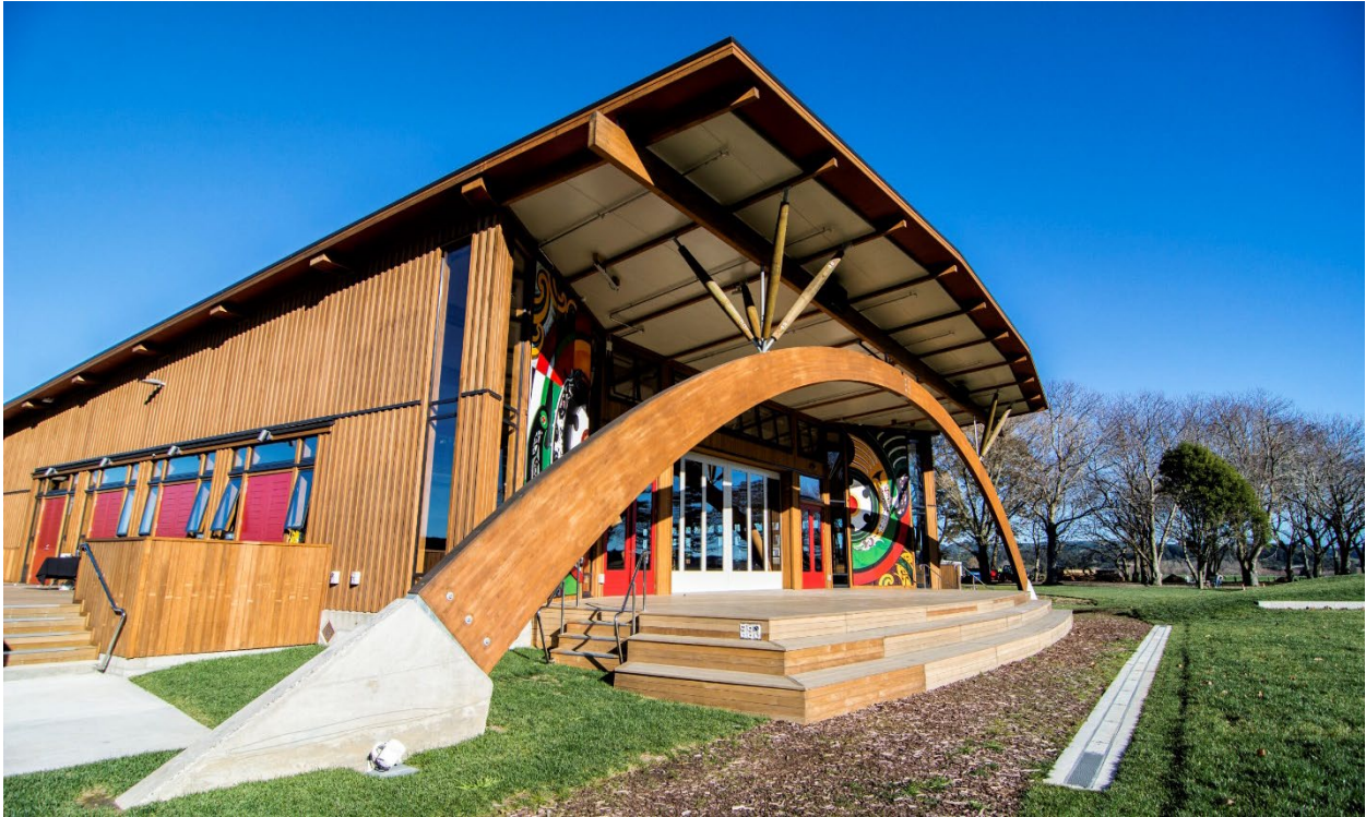
Figure 17. Te Kura Whare's exterior glulam structure, courtesy of the International Living Futures Institute.
