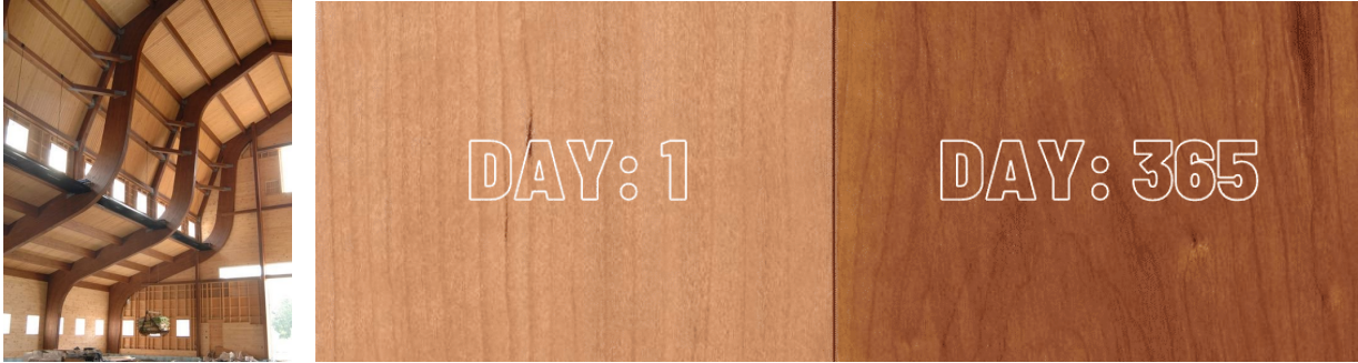
Figure 4 (left). Reverse curved arches created with FSC certified glulam for the Silver Mountain Hay Barn in Millerton, New York, courtesy of Unalam.
