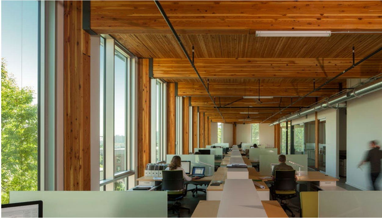
Figure 8. The Bullitt Center's top floor's engineered wood columns and beams, courtesy of bullittcenter.org.
