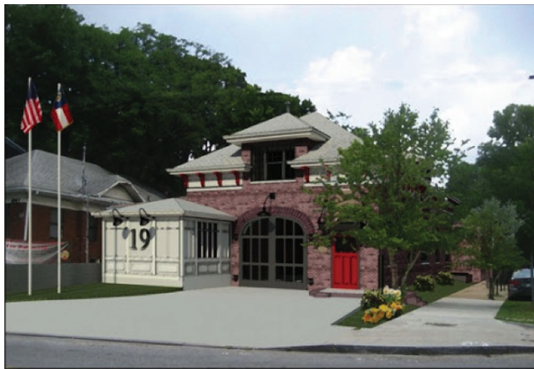
Fire Station 19 Renovation 1063 N Highland Ave
