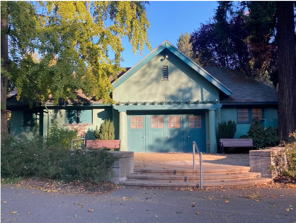
Figure 13: The Ankeny Street comfort station is the only building inside the park's original footprint, November 2022
