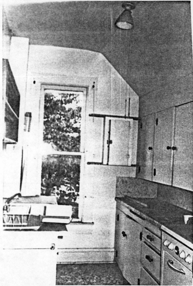
second floor - kitchen looking north
