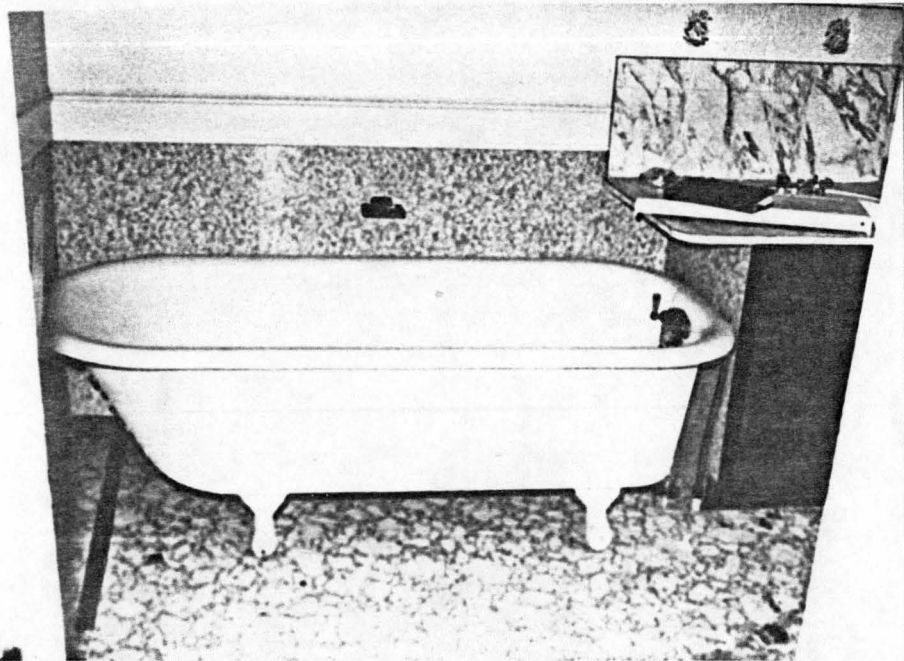
second floor - bath looking west
