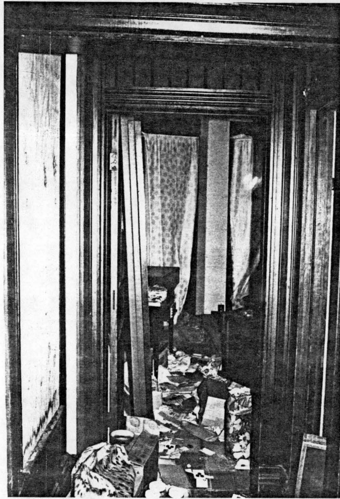
first floor - hall looking south
