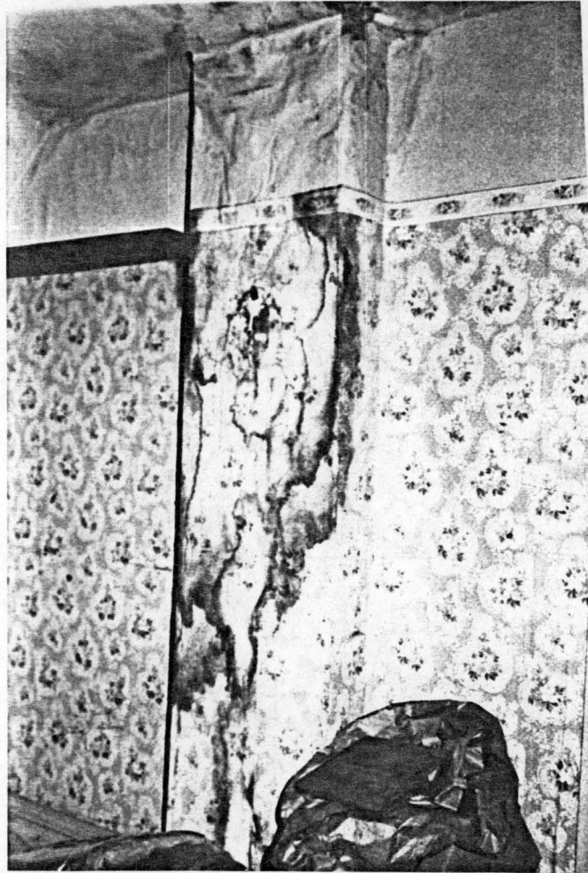
second floor - south bedroom chimney detail
