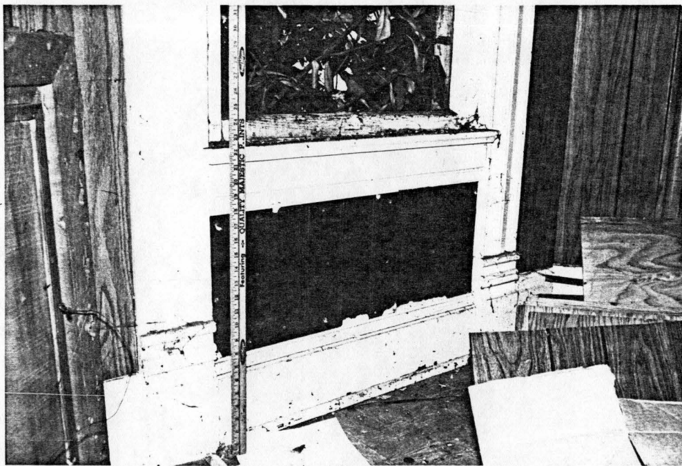
first floor - dining room - detail
