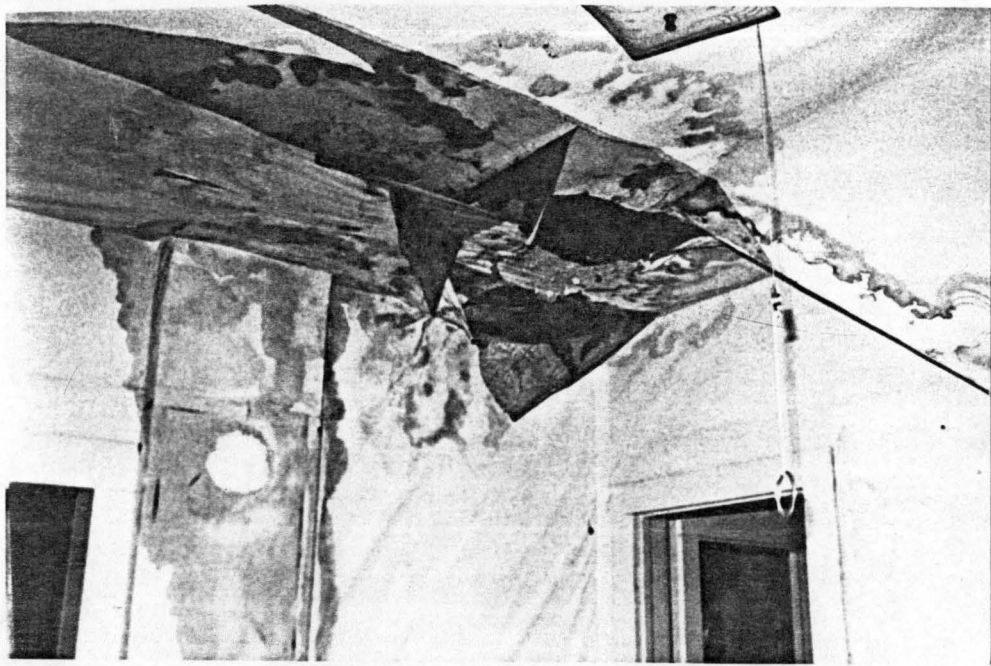
second floor - east bedroom - ceiling detail
