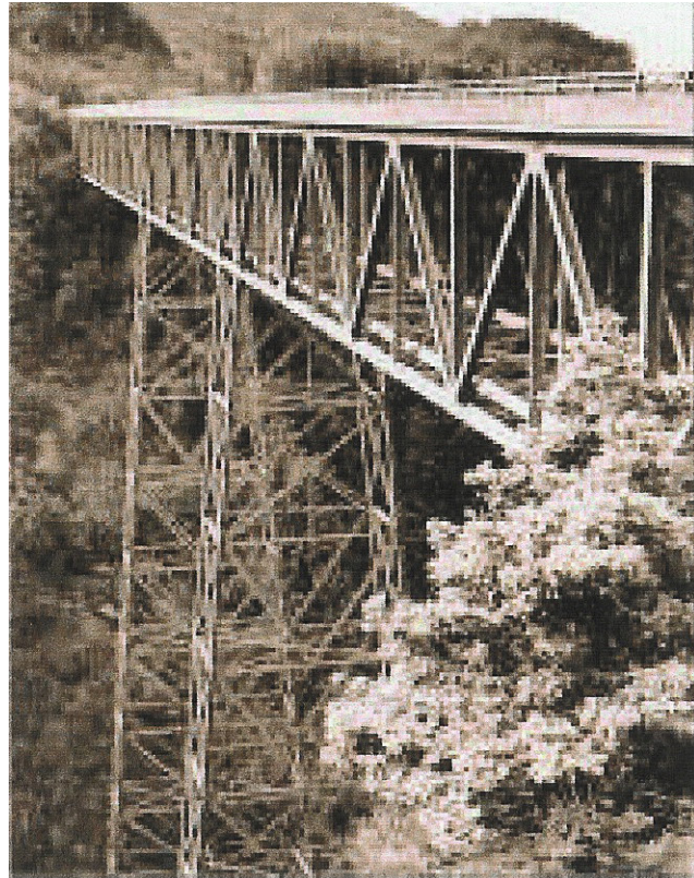
Thomas Creek Bridge U.S. Highway 101, near Brookings
