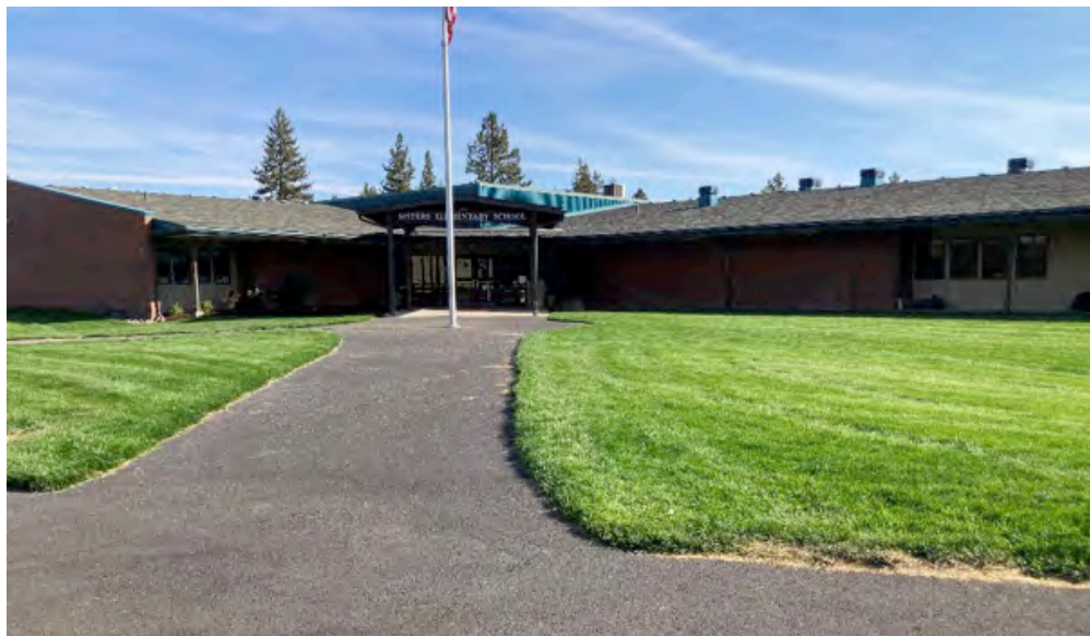
Figure 3: Sisters Elementary School entrance.
