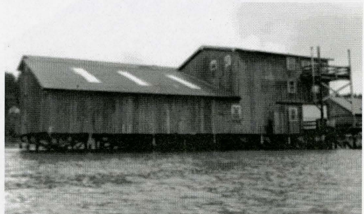
Figure 5: Northeast corner of Alderbrook net shed Photo by author, February 2012.
