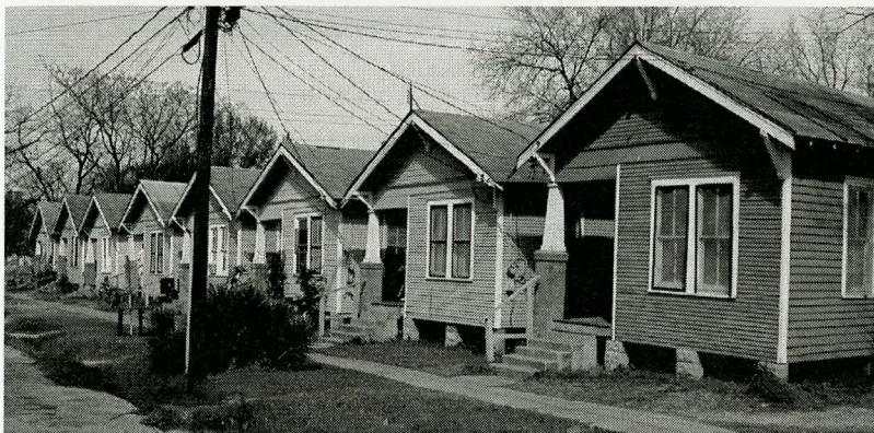
Figure 8. Residential Block Lined with Row Houses
