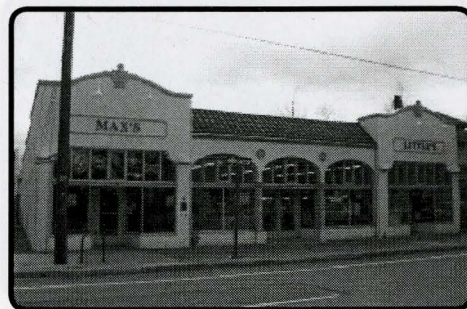
Figure 5: Thompson-Roach Building, Photo courtesy of Sarah Steen.
