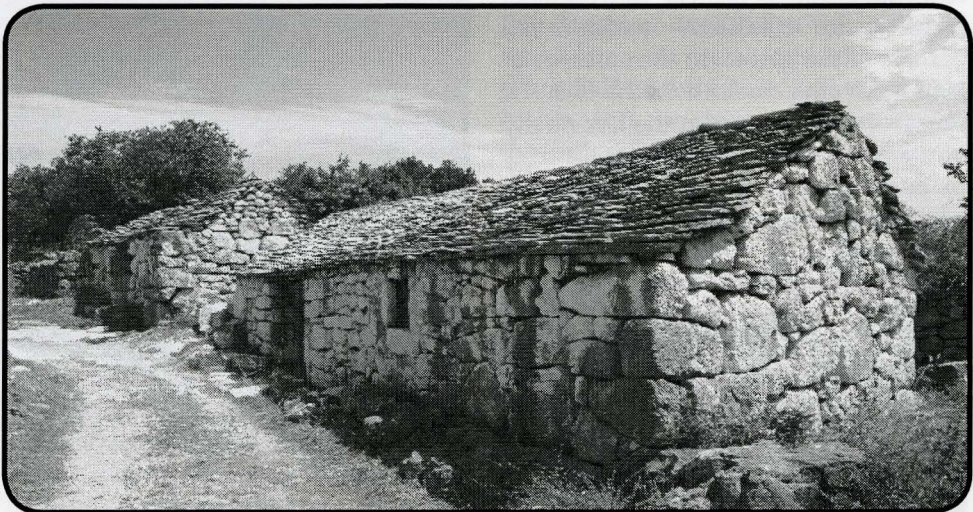
Figure 3: Typical vernacular limestone dwellings on central Dalmatian coast. Photo courtesy of Kingston Heath.
