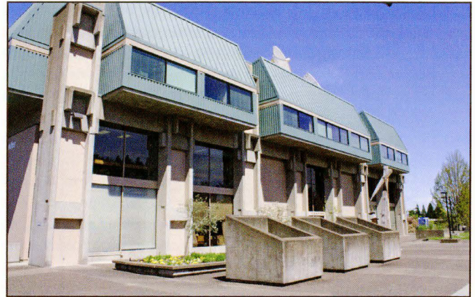
Image 2: Center Building at Lane Community College Main Campus. Light wells are in the foreground, providing light to the lower level beneath. (Photo: David Casteel)
