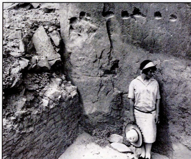
Image 1: Adobe wall construction consisting of a rubble and adobe core with dressed sandstone exterior. Layers of plaster wall coating can be seen on the rear wall with remnants of roof beam seats.
