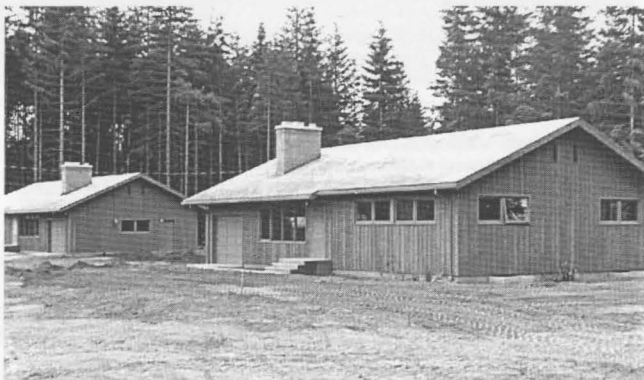
House #1228, construction completed, front and side elevations, view northwest, B/W, JUN 59. Note: House #1053, construction completed, at left.
