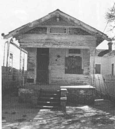
Operation Comeback shotgun house in the Holy Cross neighborhood. Photo: Helwick
