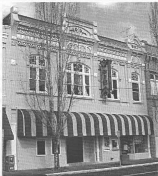
The Straney-Moore Livery stable in its reincarnation as the Pix Theatre. Recent work exposed two long lost cast-iron columns at the center of the storefront.
