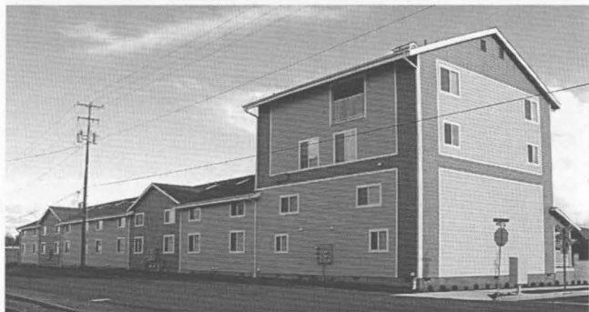
The Jefferson Lofts apartment complex, completed in 2005. The core of the structure is a seed warehouse, built circa 1912. Photo: Neiderer
