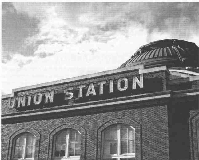
Built in 1911, the Reed and Stem designed Union Station in Tacoma is now home to a federal courthouse. Photo: Donaghy
