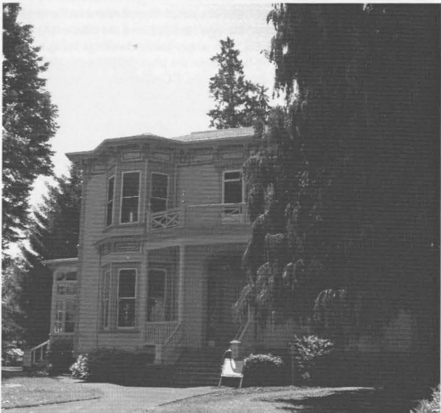
The 120-year old Collier House on the University of Oregon. Built in 1886 by a professor at the University, the structure has recently endured a strenuous mold abatement process. Photo: Donaghy
