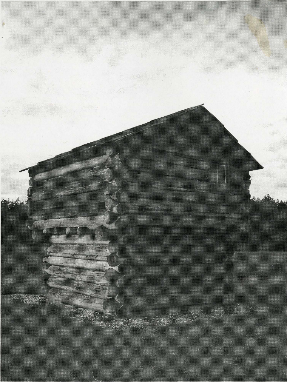
The block house at the Jacob Ebey House on Whidbey Island, Washington. This photo was taken as a part of the Building Recordation class taught by Don Peting during Winter 2006. Photo: Donaghy
