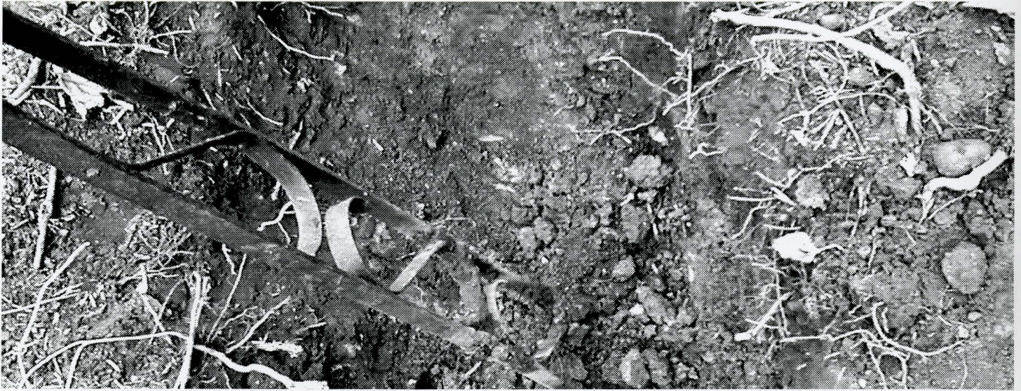
Excavation on the Normal Gate in progress. Approximately five feet of the structure was buried.
