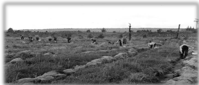
In the 1930's most of the project area was tractor furrowed and planted with jack pine. The above photo shows a CCC crew planting the present-day project area. Note the thick sod layer, barrens landscape, and fire-scarred snags
