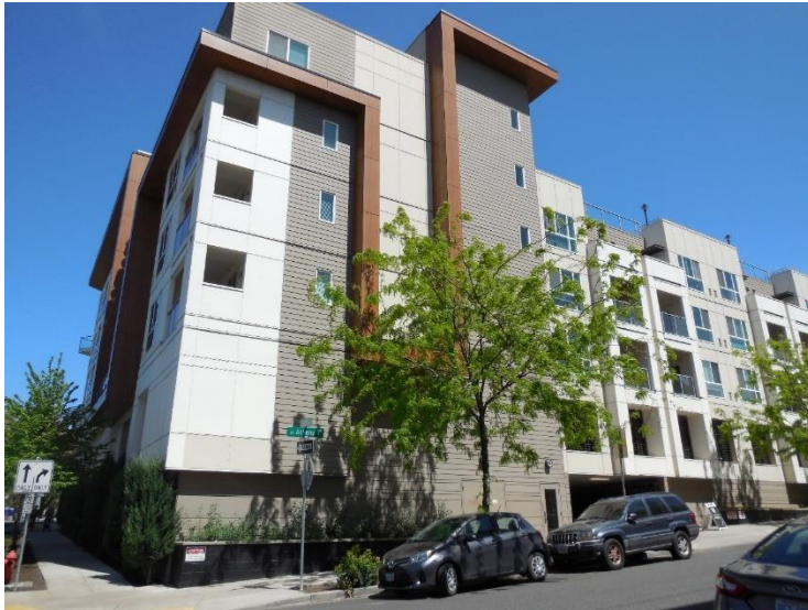
Figure 15: 1250 SE Burnside Street. Photo by author.
