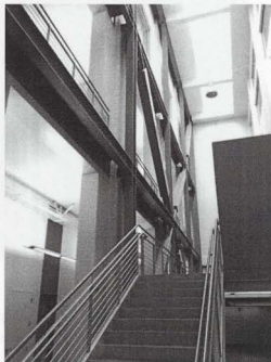
Figure Nineteen: Lincoln Hall restored light wells. Photo by author.
