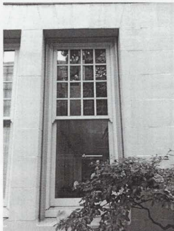
Figure Eighteen: Lincoln Hall high performance windows (replicas of original wood windows). Photo by author.
