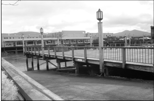
Boat ramp at Quatat Park
