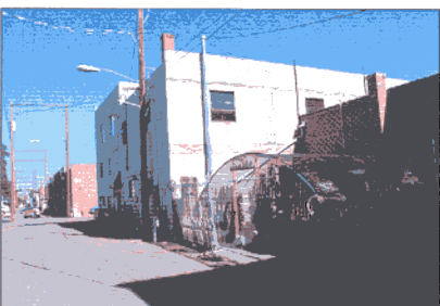
Alley behind 6th Street
