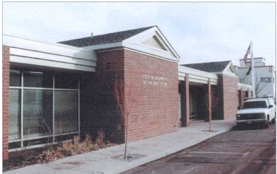
Redmond Municipal Court Building
