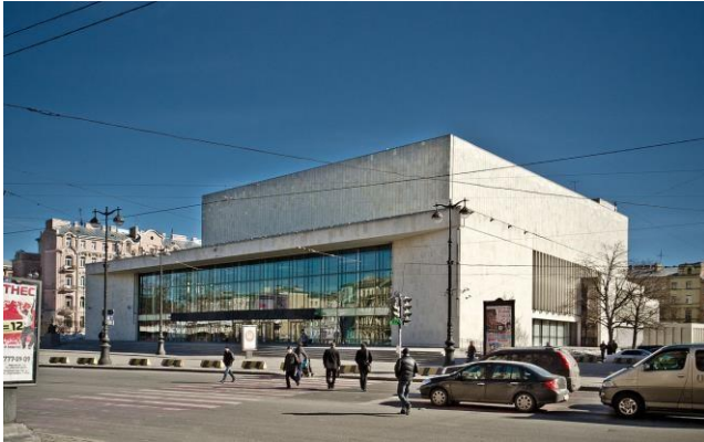
Fig. 2 Bol'shoi kontsertnyi zal Oktiabr'skii (The October Big Concert Hall (BKZ)). The Concert Hall was erected in place of the “Greek Church” in the Greek Square. It opened in October 1967, inaugurating the fifty-year-anniversary of the October Revolution.
