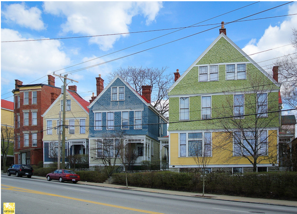
FIG. 6 Missing Middle Housing in Walnut Hills by Opticos Design, cc Sightline Institute.
