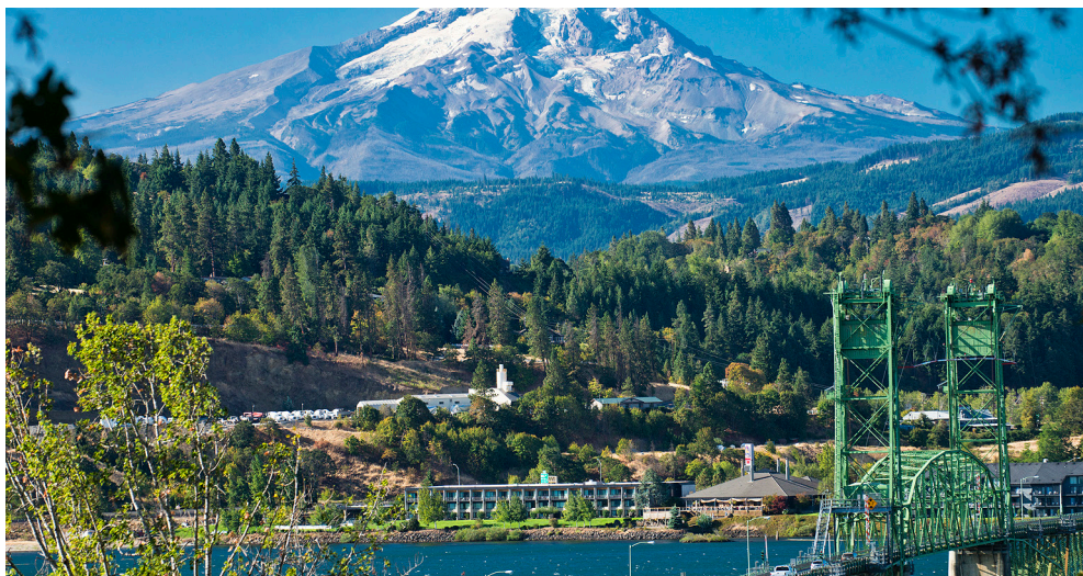
FIG. 4 Hood River Bridge.
